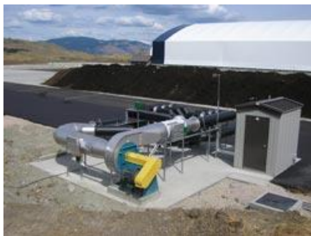
Picture 3 (Uncovered aerated static pile)
