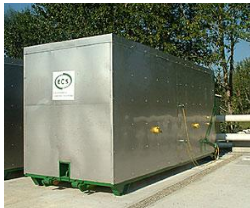
Picture 2 (Stainless steel & concrete in-vessel compost system)
