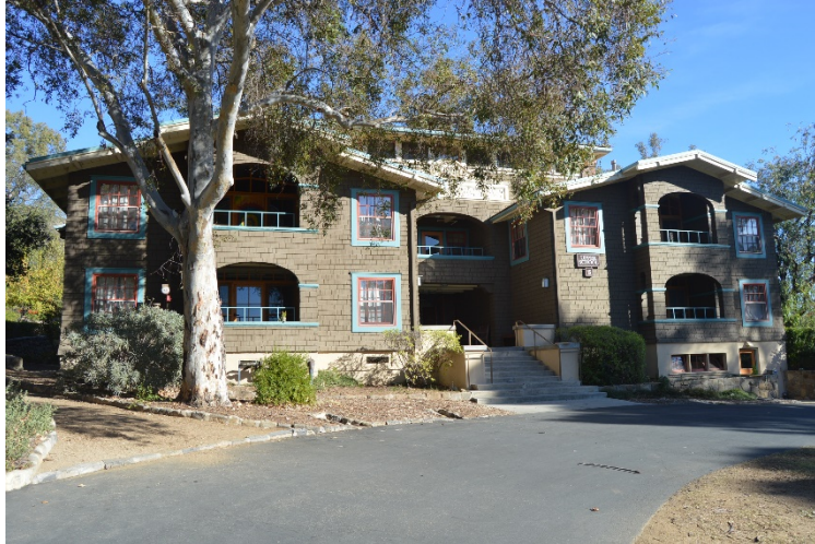
Upper School Dormitory, view looking east
