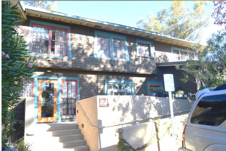
Dodge Annex, view looking southeast
