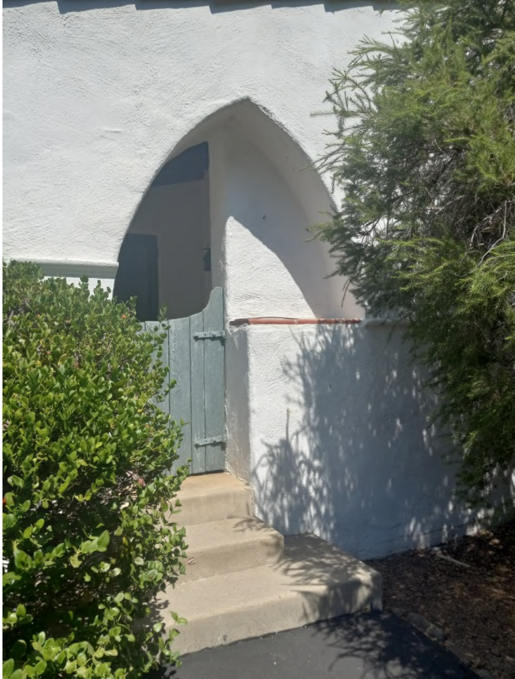
Photograph #13 Property at 3935 Thacher Road South elevation, detail of arched doorway
