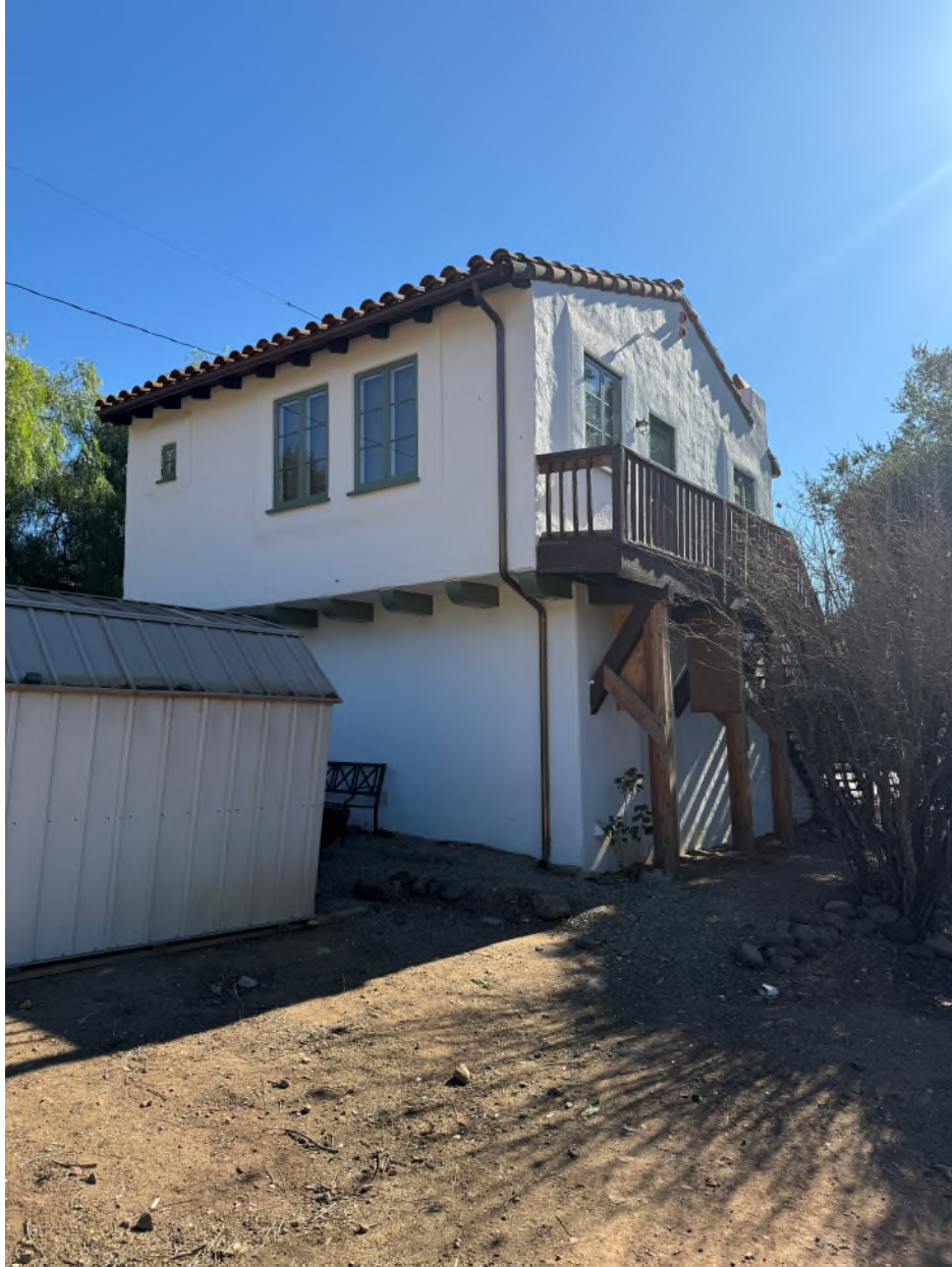
Photograph #26 Property at 3935 Thacher Road North elevation of the garage (Looking SE)
