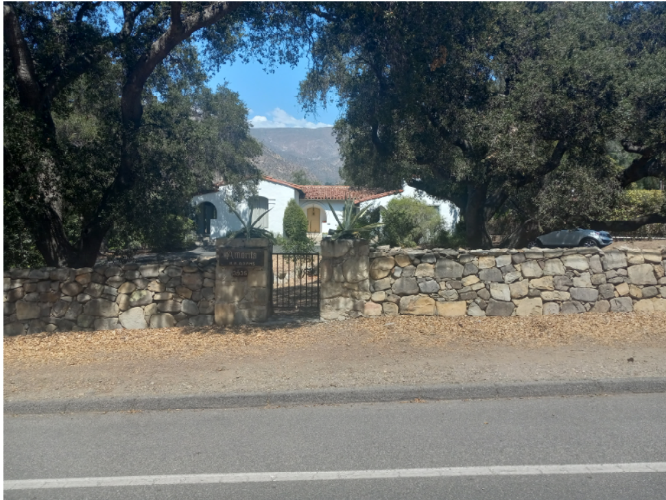
Photograph #7 Property at 3935 Thacher Road South elevation of house (Looking north)
