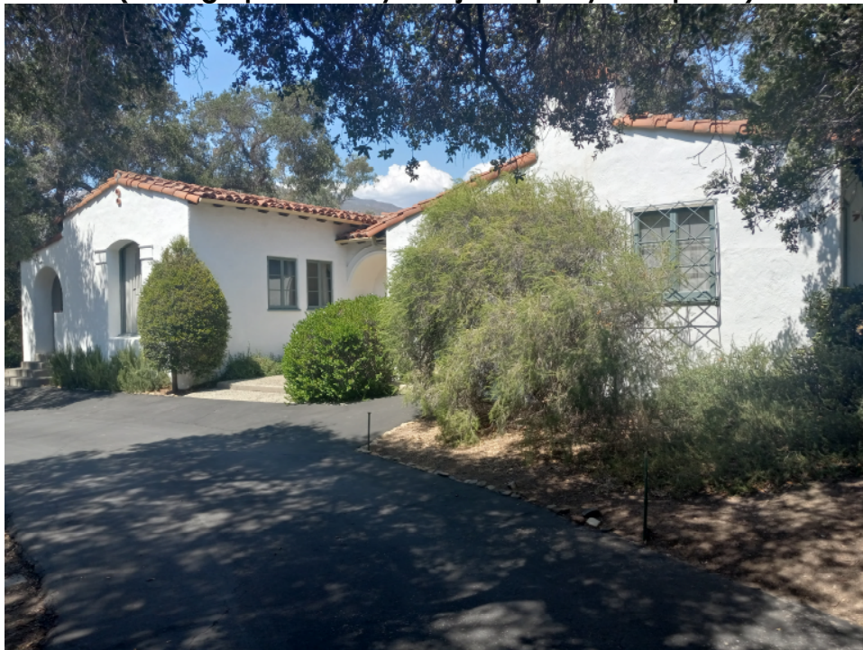
Photograph #9 Property at 3935 Thacher Road South elevation of house (Looking NW)
