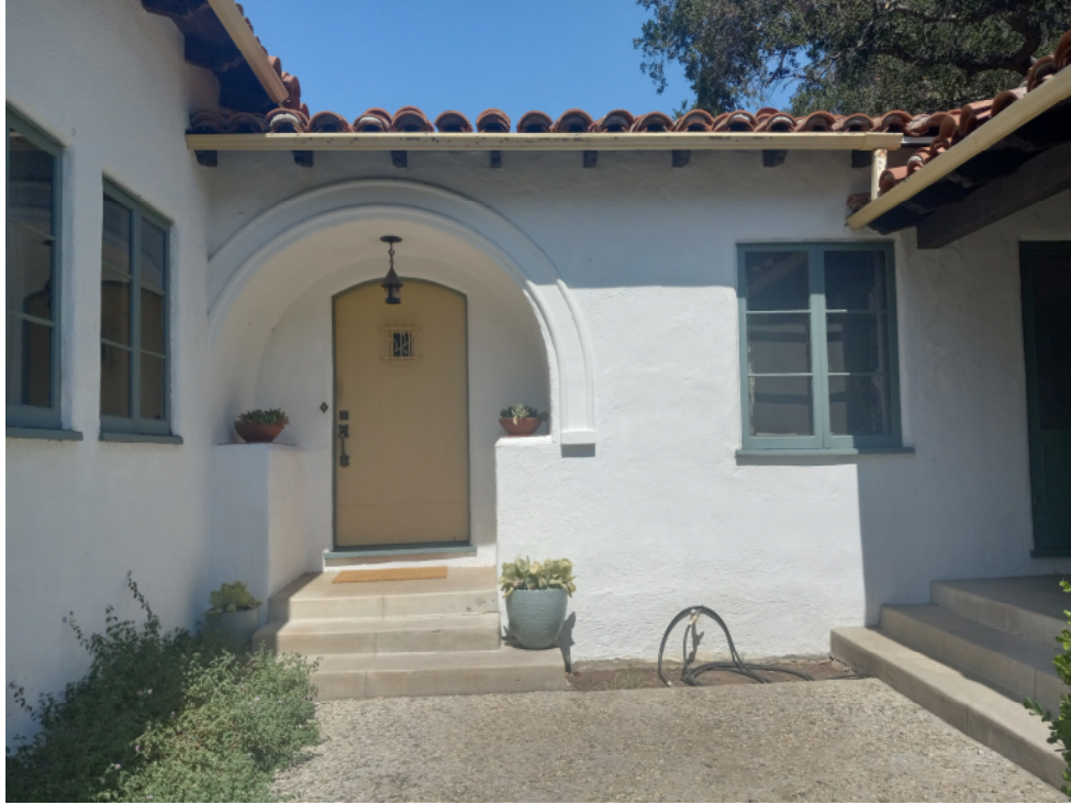
Photograph #10 Property at 3935 Thacher Road South elevation of house (Looking north)
