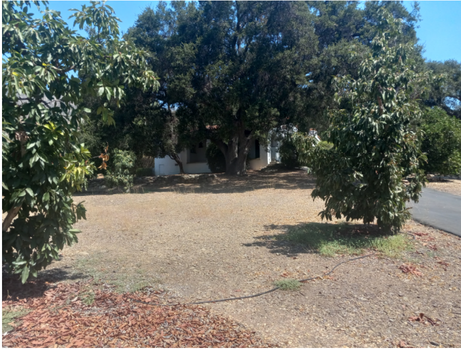
Photograph #18 Property at 3935 Thacher Road West elevation (Looking NE)
