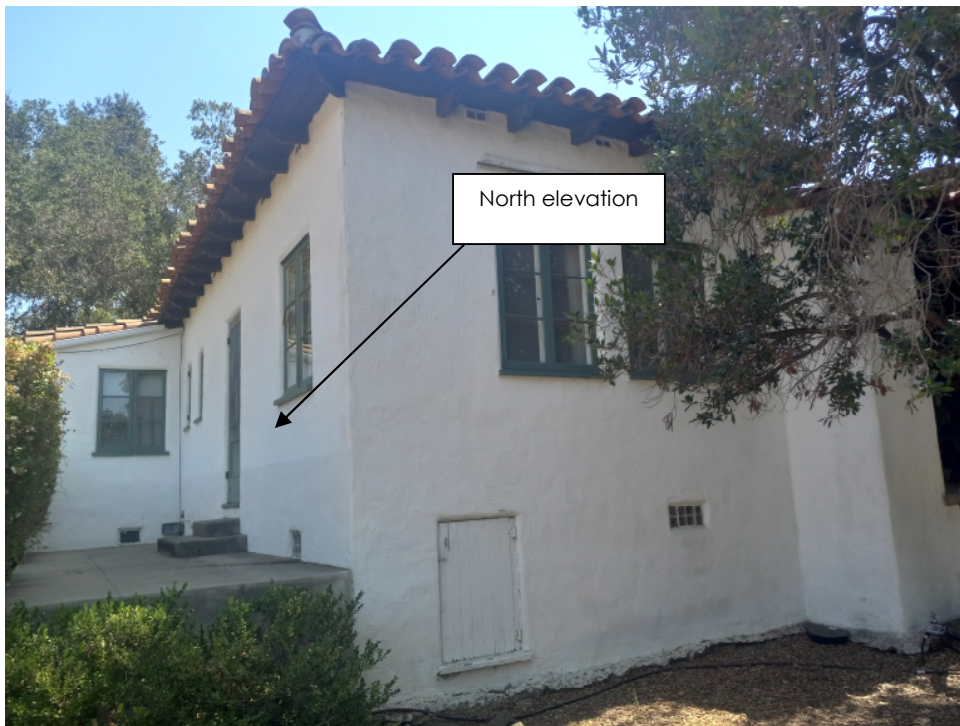
Photograph #15 Property at 3935 Thacher Road West of north elevation (Looking east)
