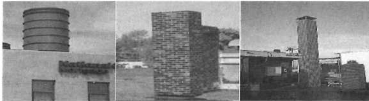
Examples of Roof-Mounted Wireless Communication Facilities (ADD. ORD. 4470 – 3/24/15)
