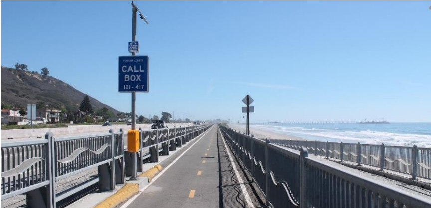
This Multi-Modal Route (N1) includes a path constructed by Caltrans as part of the Ventura to Santa Barbara Highway 101 HOV project.
