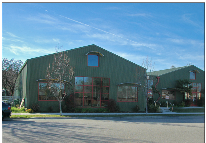
Illustrative Photo of Industrial Buildings with pitched roofs
