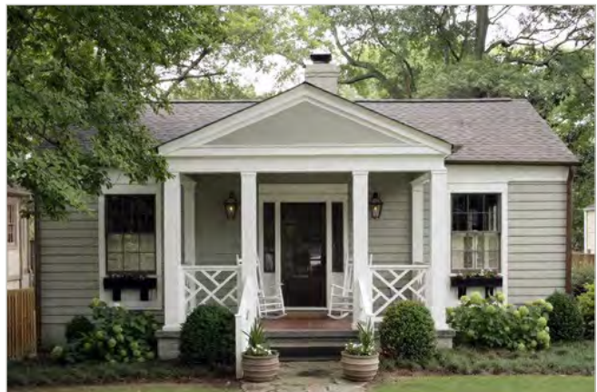
Image 6.8. A porch addition that uses materials and design matching to the existing home.
