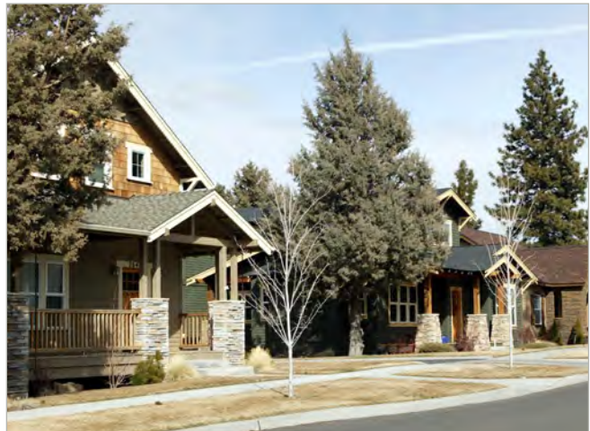
Image 6.7. Entrances to residences are clearly identified by projecting forms such as porches.
