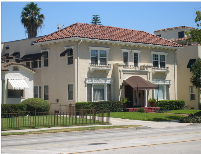
Illustrative Photo of a small apartment building.
