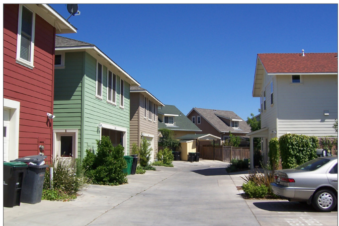
Accessory buildings have alley-facing windows.
