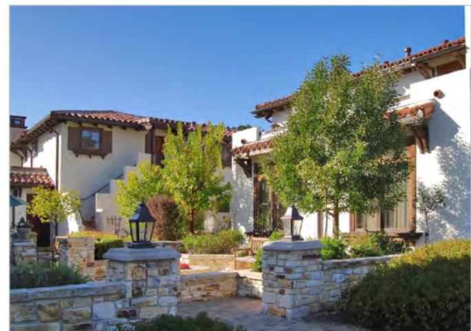
Image 6.5. Multi-family residential development designed as a group of smaller residential buildings.
