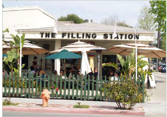
Image 6.3. Building that retains the original character of a gas station while adapted for a new commercial use.
