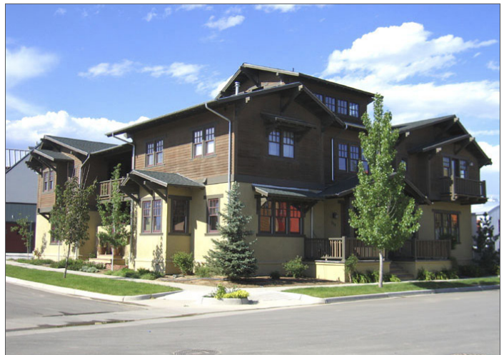
Illustrative Photo showing a Quadplex, allowed as a 3 story in the Residential/Mixed Use zone only.
