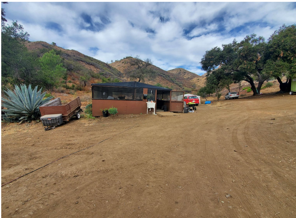
View looking west at Structure No. 5.
