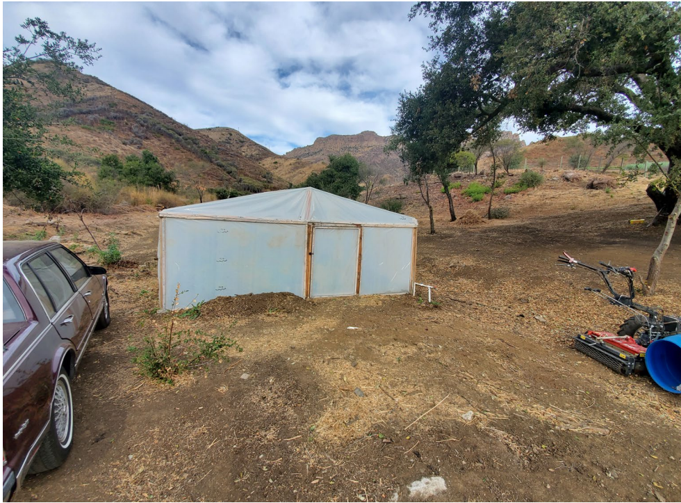
View looking northwest at Structure No. 6.
